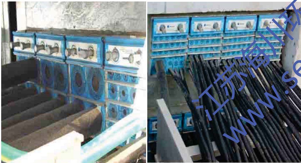
烙克赛克密封 Roxtec sealing
